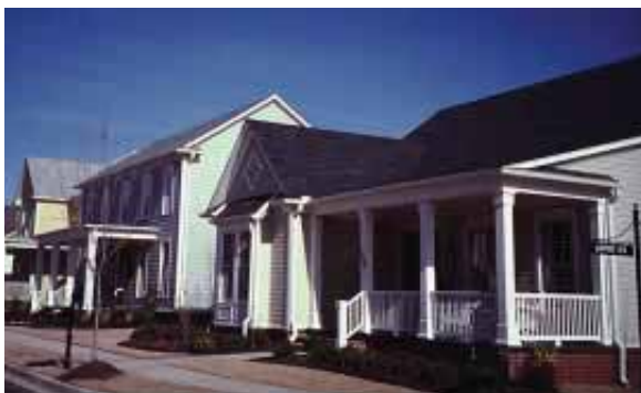
Houses in Magnolia Square use new fiber-cement siding as an acceptable alternative to wood siding.
