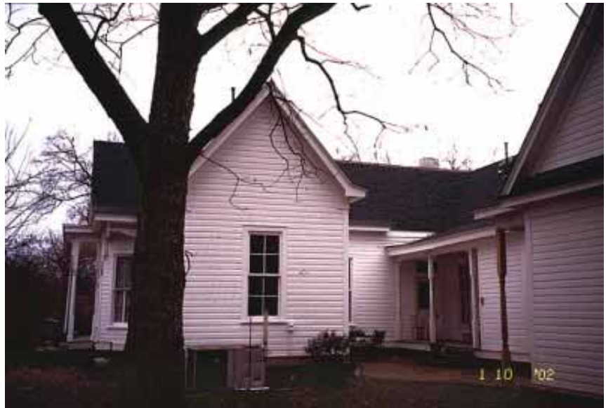
This new addition is connected to the existing house without detracting from the original primary elevation.
