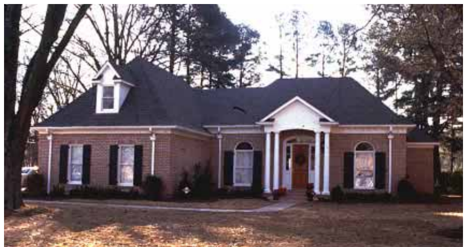
The classical portico on this new house creates a formal architectural element.
