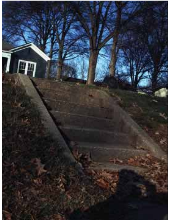
Front steps are common in the historic district.
