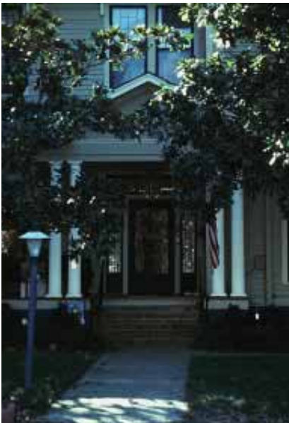
This entry portico helps define the architectural style of this home and focus attention on the original door, sidelights and transom.
