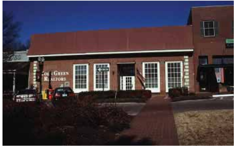
The size and proportion of the windows are not compatible with the surrounding buildings.
