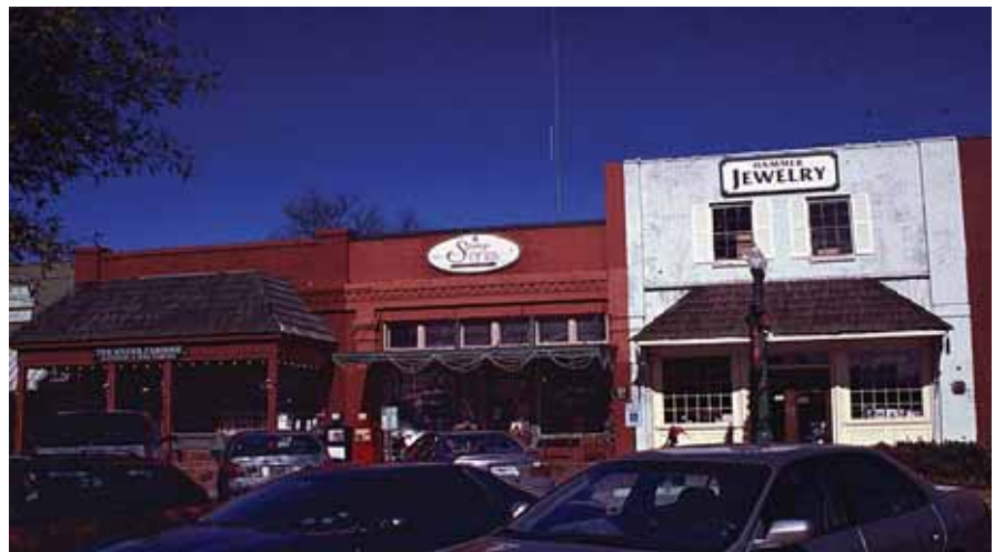
Collierville has a variety of original and retrofitted storefronts
