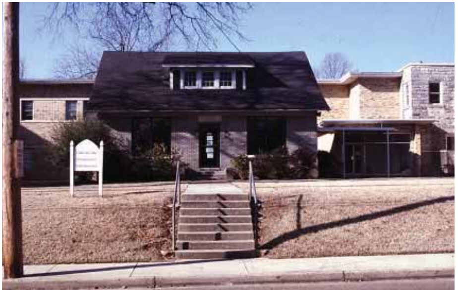
The owners of this building have preserved its dormer window and other residential features, even though it is now used as an office.
