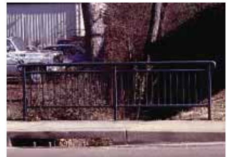
The historic district has nice streetscape elements including guardrails like this one.
