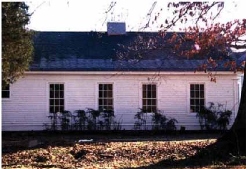
The regular shape and rhythm of these windows adds to the character of the building.
