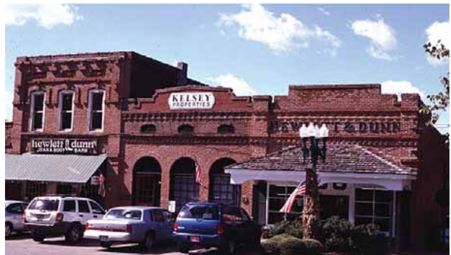
These historic structures have highly decorative brick corbelling, cornices and copings.
