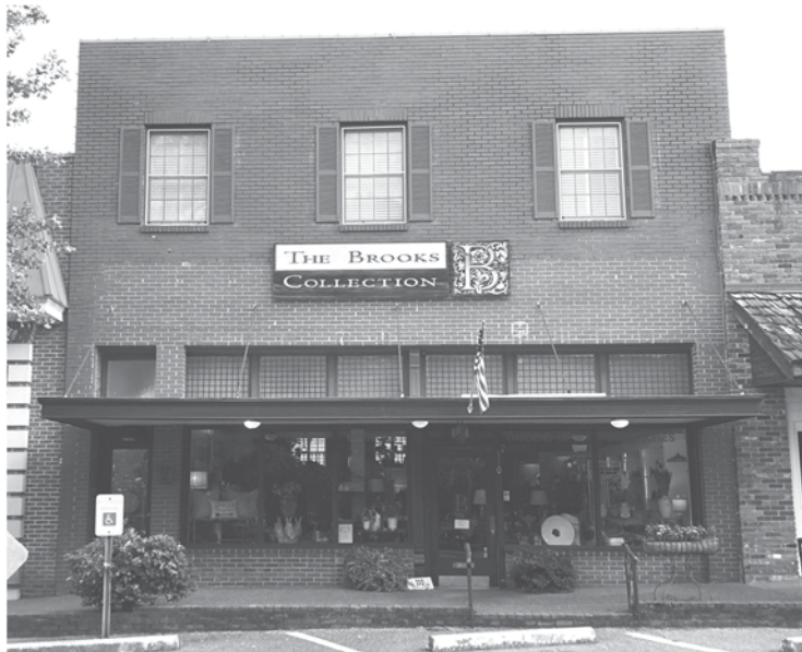
Flat metal canopies such as this one are appropriate on commercial storefronts.
