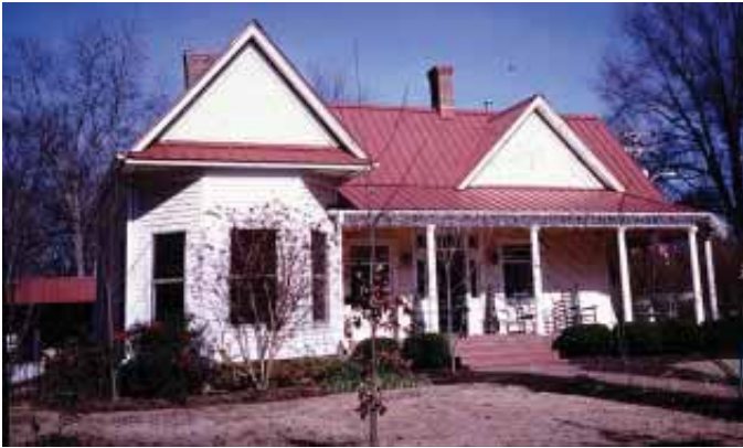
Historic style roofing material, such as this standing seam metal roofing, is appropriate on certain houses.
