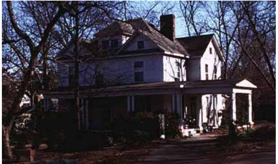
Complex forms on new and old homes often include many different projections, indentions, and rooflines.
