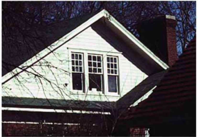
These windows still have their original upper sash intact.
