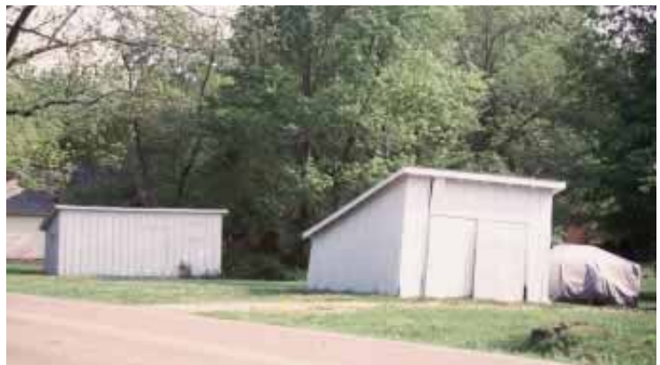
Sheds and other historic outbuildings reflect the village heritage of Collierville and should be preserved.
