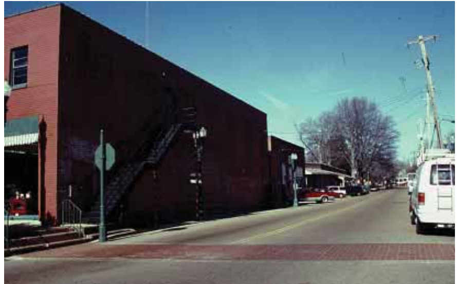
The side elevation of this building faces a significant entry into the Town Square and could be a better architectural element for the area.
