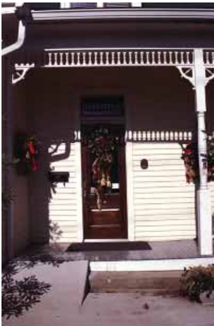
This door has maintained its original configuration, including its transom window.
