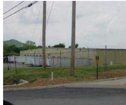
Loading area unshielded from public street
