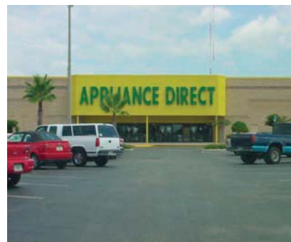
Surface parking areas between street and building
