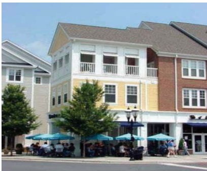
A mix of smaller shops with larger commercial uses
