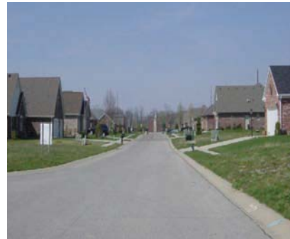
Curb and gutter and other urban improvements
