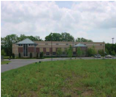
Storage area screened from public street
