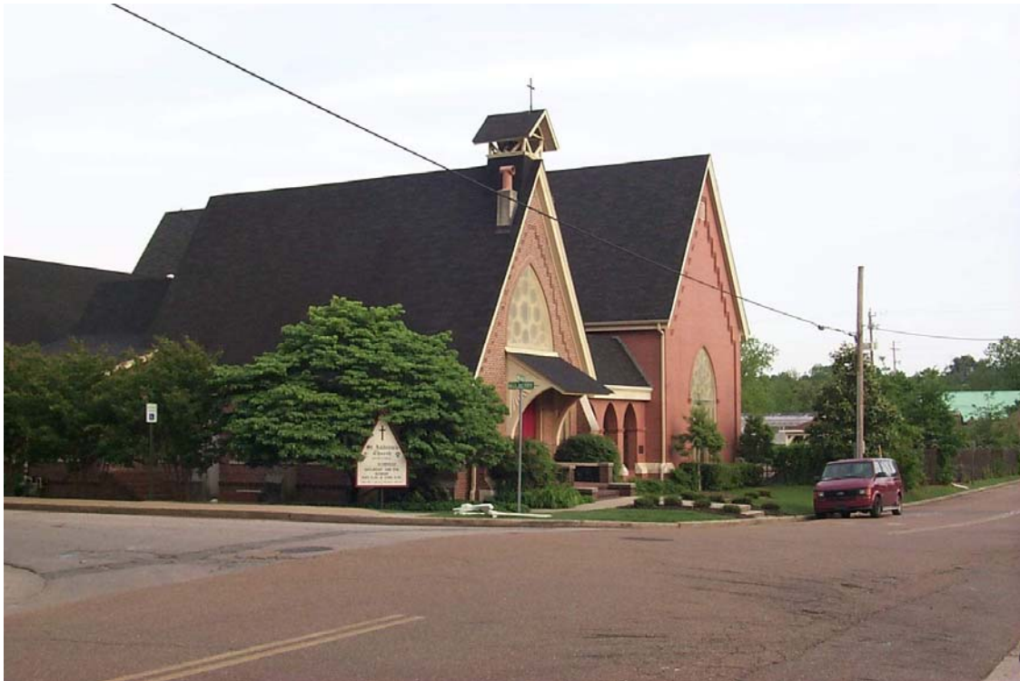
Influenced by the Gothic Revival style, St. Andrew's Episcopal Church, constructed in 1890, possesses a steep gable roof with wide projecting eaves and a small, cupola-like bell cap steeple.
