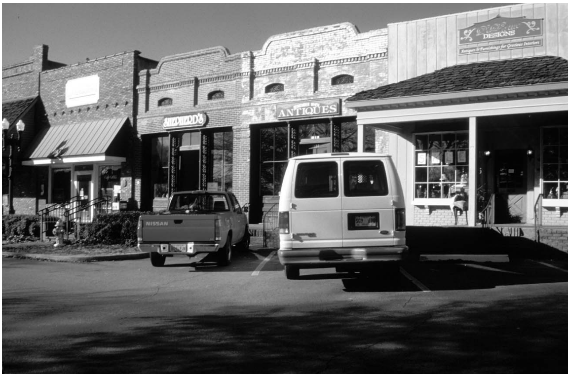
The commercial buildings encompassing Collierville's Town Square provide a strong identity not enjoyed by other communities in the region. While most of the buildings have been well-maintained and have an attractive appearance, many have undergone inappropriate alterations, such as canopies that are not historically correct.
