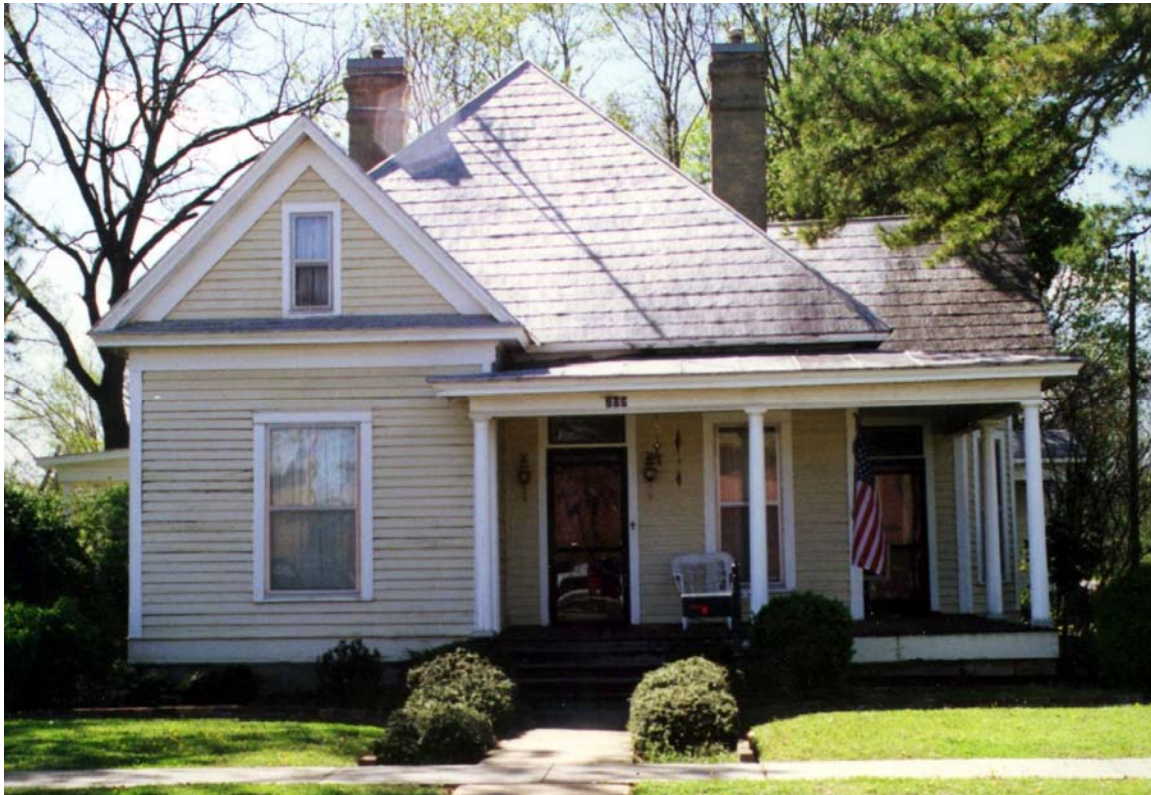
This circa 1900 cottage is typical of those found in the historic neighborhoods surrounding Collierville's Town Square area. Common features include the clapboard cladding, steeply-pitched roof with multiple gables, raised foundation, vertically oriented openings, and wrap-around front porch.
