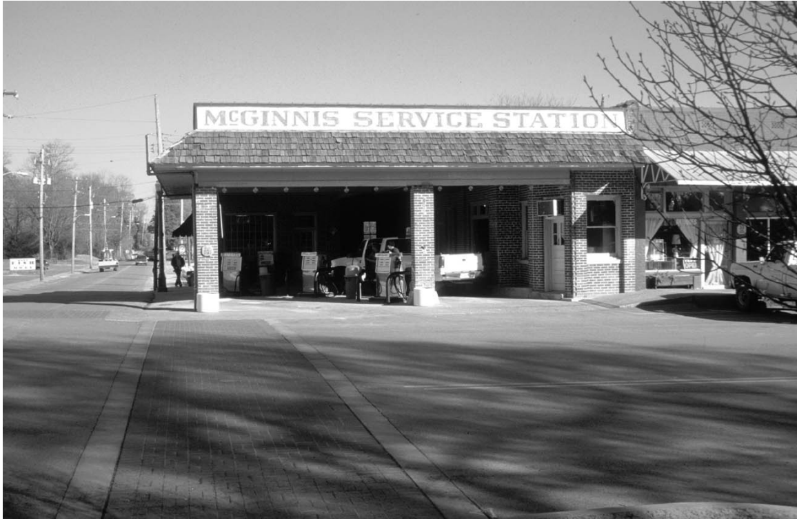
The McGinnis Service Station, located on the eastern side of the Town Square, is highly-significant to the history and the character of the Square, and its preservation is an important goal.
