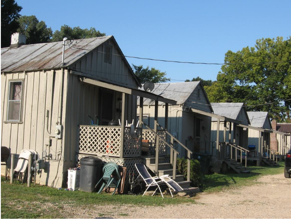
Row of Shotgun houses on E. South Street.
