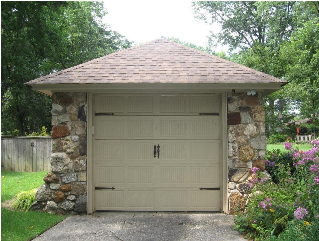
Original stone-veneer garage at 232 E. Poplar Ave. (SY-30498).
