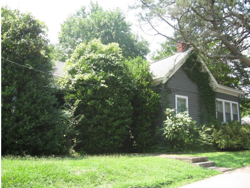
Jack Dudney House, 90 W. Poplar Avenue (SY-30497)
