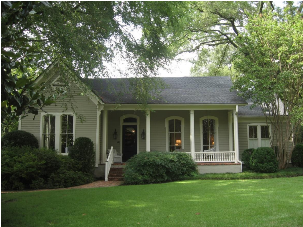
Gabled Ell dwelling at 260 N. Rowlett Street (SY-30361).
