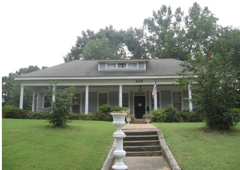
John W. Thomas House, 245 W. Poplar Avenue (SY-30530)
