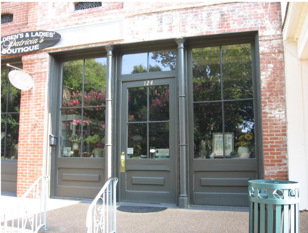
Example of an original storefront with cast iron at 124 E. Mulberry Street.
