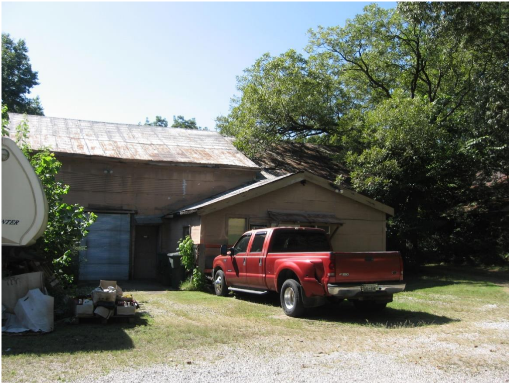
Ice plant building at 166 Mills Street.
