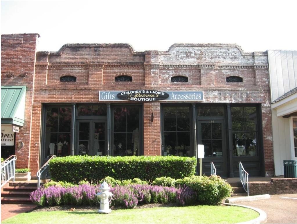
One-story commercial buildings at 122-124 E. Mulberry Street (SY-30239).
