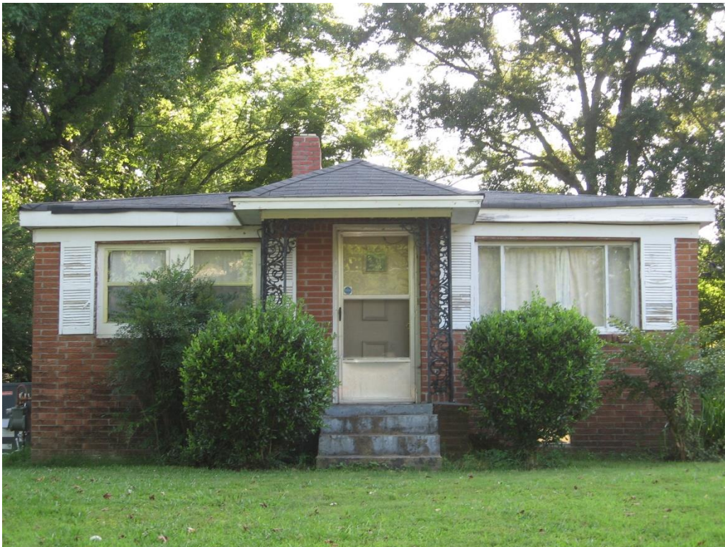
Minimal Traditional style dwelling at 4201 Bailey Station Road, (SY-24913).
