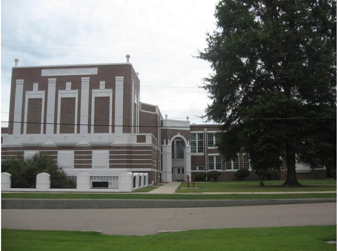
Collierville High School, 146 College Street (SY-30290)
