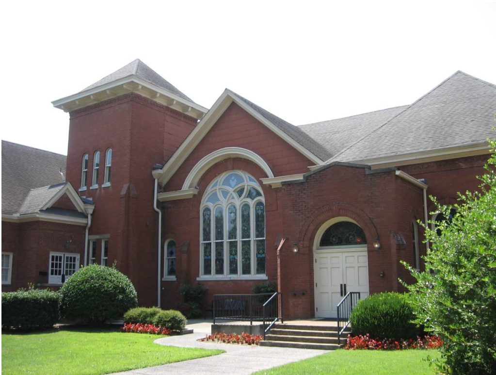
Collierville United Methodist Church at 104 N. Rowlett Street (SY-30288).
