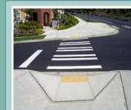
Road & Sidewalk Improvements
