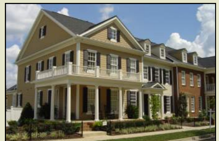
These townhouses contain a mix of roof forms
