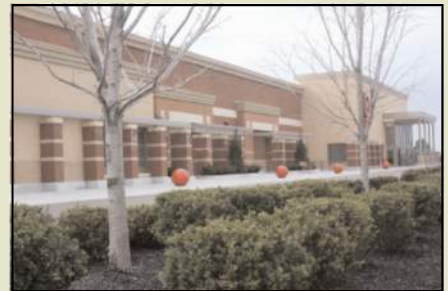
Details such as colonnades with keystones and pergolas help add human scale to long facades
