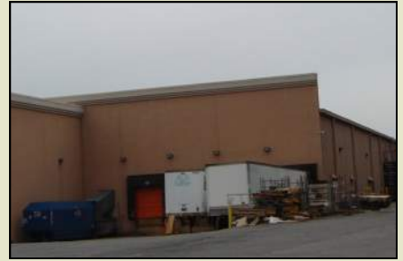
A loading and service area with no screening
