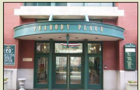
Canopies at entries are typical for large buildings
