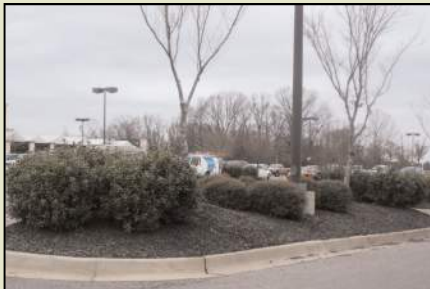
Space islands no more than 15 spaces apart
