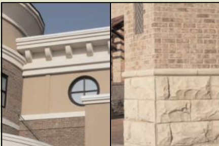
Appropriate uses of simulated wood trim and EIFS accent (l) and textured simulated stone (r)
