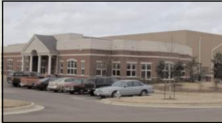
This industrial building uses changes in plane, materials, and a stepped back height to reduce impact of its mass where visible from public
