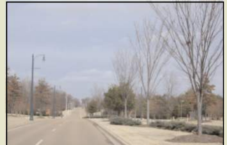
Orderly placement of lighting and landscaping
