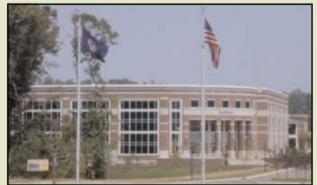
Color combinations & texture of cast stone and masonry help to give a human scale to this facade
