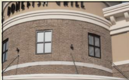
Cornices, belt courses, and changes in materials, combined with changes in massing, are encouraged
