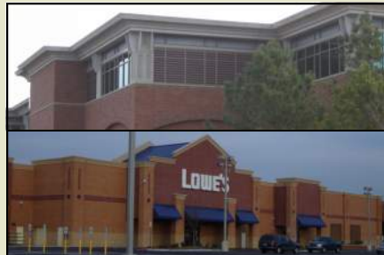
Mechanical units screened with architecture
