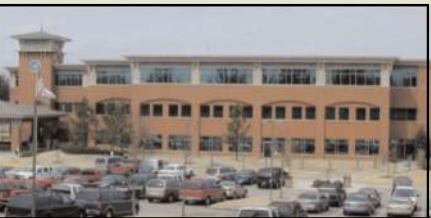
A modern example of façade articulation through bay divisions and horizontal bands
