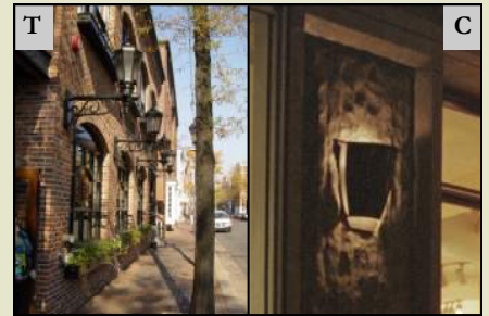
Acceptable shielded wall fixtures
