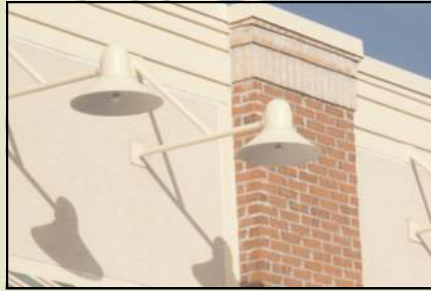
Gooseneck fixture with bulb exposed
