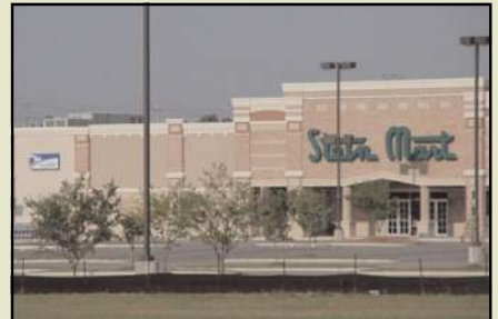
Mechanical units are visible above parapet
