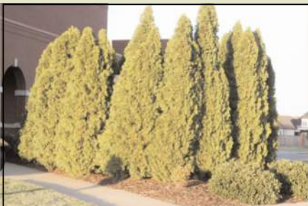
A transformer screened with evergreens
