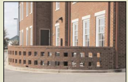
Mechanical screen wall that matches building
