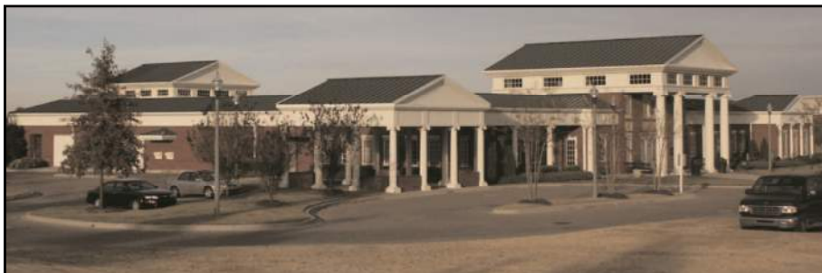
The roof forms on the Town Hall effectively screen the building's rooftop equipment.
