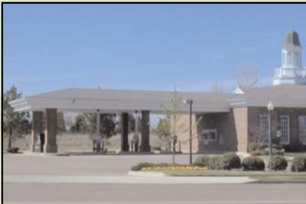
Match columns and cornice to building
