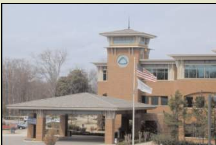
Towers can add interest while breaking up mass
