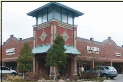
Architectural features provide interest at corners
