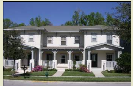
Triplex with porches, columns, and exposed eaves
