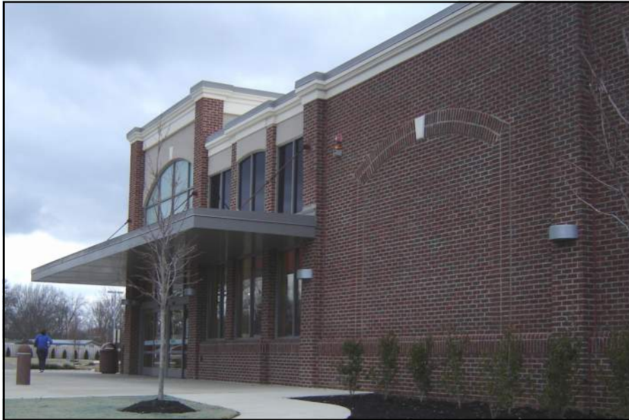
Human scaled details such as canopies, cornices, belt courses, water tables, bay divisions, win-
