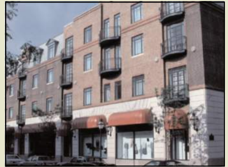
This hotel uses a stone base and two colors of brick, combined with a single mansard roof and colored awnings, to reduce its scale
