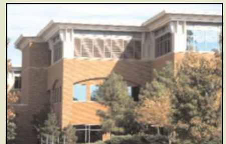
Rooftop units integrated into the architecture
