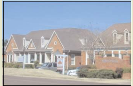
A mixed hip and gabled roof containing dormers
