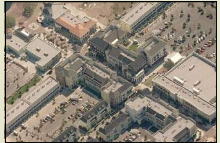
Buildings oriented to the street with rear parking
