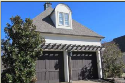
Garages with decorative doors, lights, and pergola
