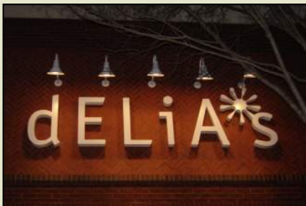
Appropriate gooseneck exterior lighting
