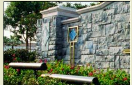
Kim lighting illuminating signage
