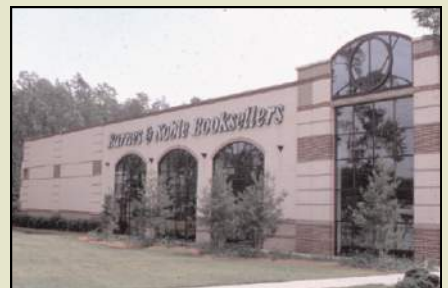
Articulate secondary facades visible from streets
