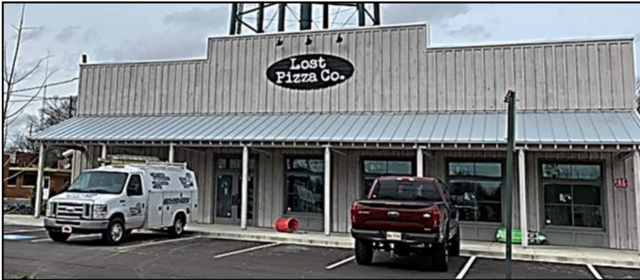
This restaurant building uses board and batten wood siding to reference exterior building materials used on historic buildings on the Town Square.
