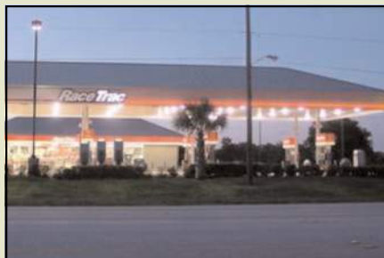
Canopy visible light fixtures creating glare
