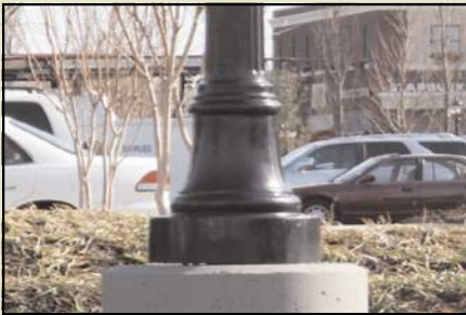
Neutral-colored pole with concrete base
