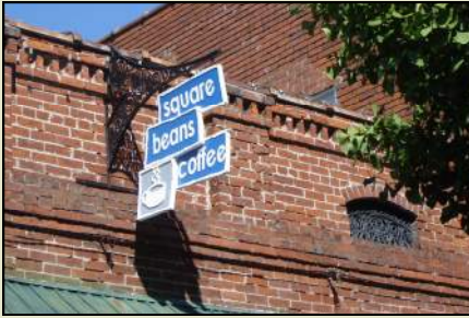
Appropriate projecting sign
